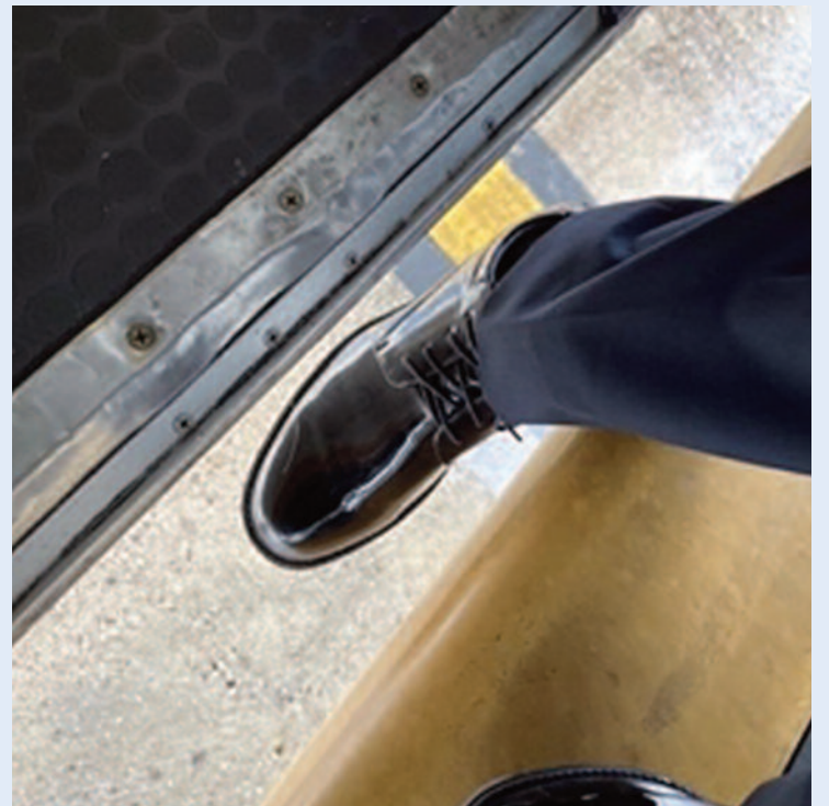
Pictured: The jet bridge not properly aligned with the aircraft.
